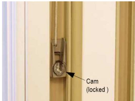
Compare clutch heights from the sill for the sash affected. They **MUST** be within 1/8" of each other or damage may occur when sash are reinstalled, adjust height as needed.
